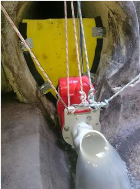
Figure 10: Variant 'Retaining wall with emergency overflow'
